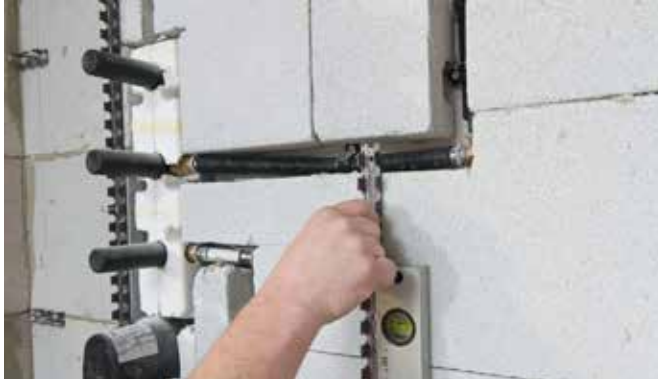
Vertical adjustment of the clip rails
