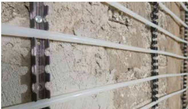
Secure fixing of the KLIMAPEX® plastic heating pipes
