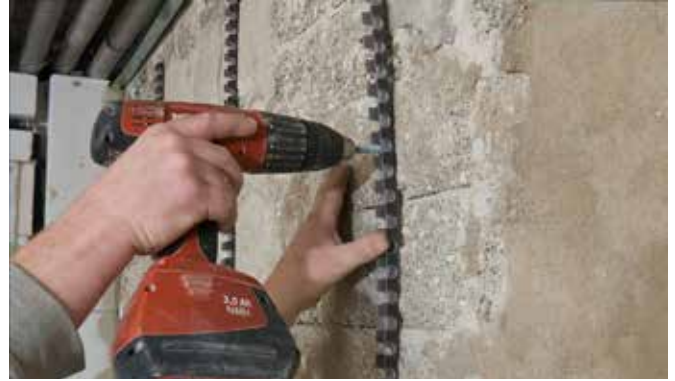
Attachment of the clip rails at a distance of max. 40-50 cm is recommended
